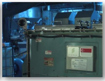
Partnering with <u>Biomax</u> Technologies in 2016, the hotel is the first in Singapore to install an in-house waste management plant consisting of a vacuum system, a grinder and dewatering unit, and a digester system to convert 1000kg of daily food waste from the hotel's 5 restaurants, 16 event venues and 677 rooms to 300kg of organic pathogen-free fertilizers within 24 hours.
