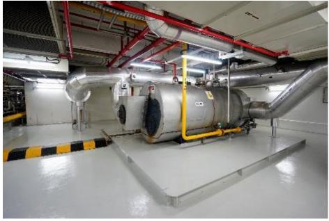
In 2011, Grand Hyatt Singapore became the first hotel in the world to install a gas-powered Trigeneration Plant to provide 30% of its electricity, as well as provide heating and cooling measures for its laundry and air-conditioning needs respectively.
